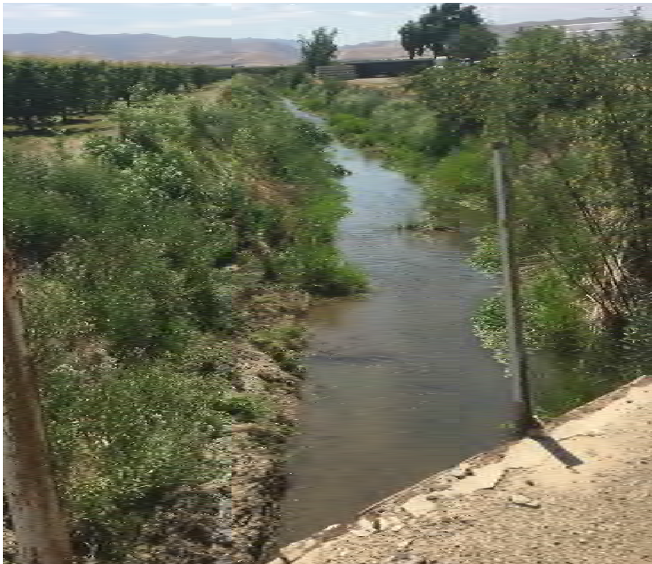
Figure 3.5-1: Lower Del Puerto Creek Above Highway 33 and Downstream of I-5
